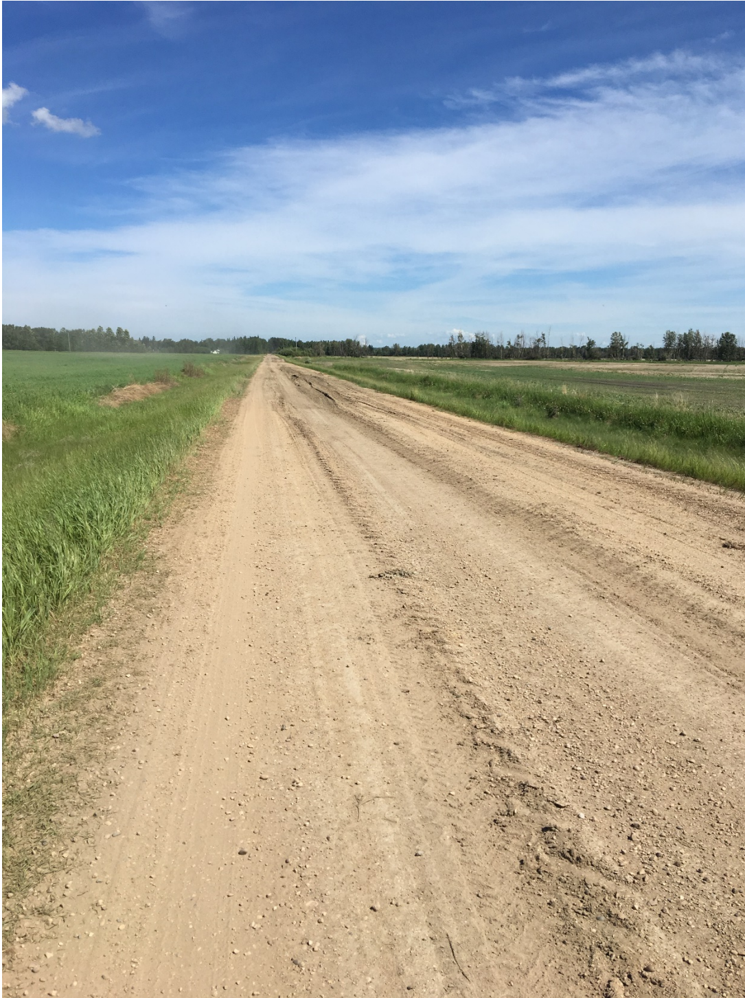
Figure 5-4 - Gravel Road in Moderate Condition (2) – Rating 3.8
