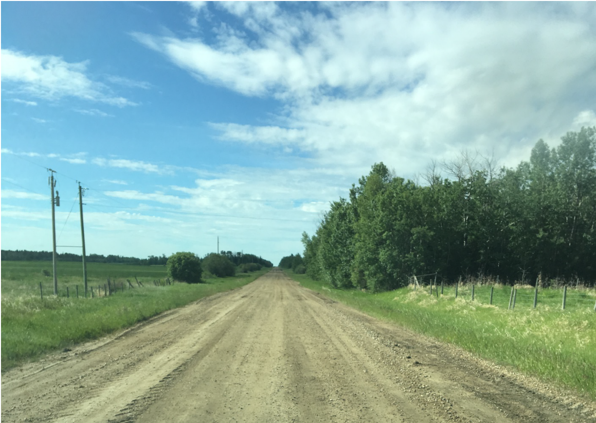
Figure 5-5 - Gravel Road in Moderate Condition (3) – Rating 4.0
