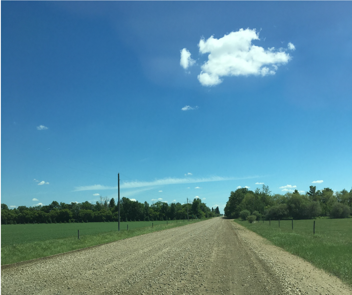
Figure 5-8 - Gravel Road in Good Condition (2) -Rating 4.8
