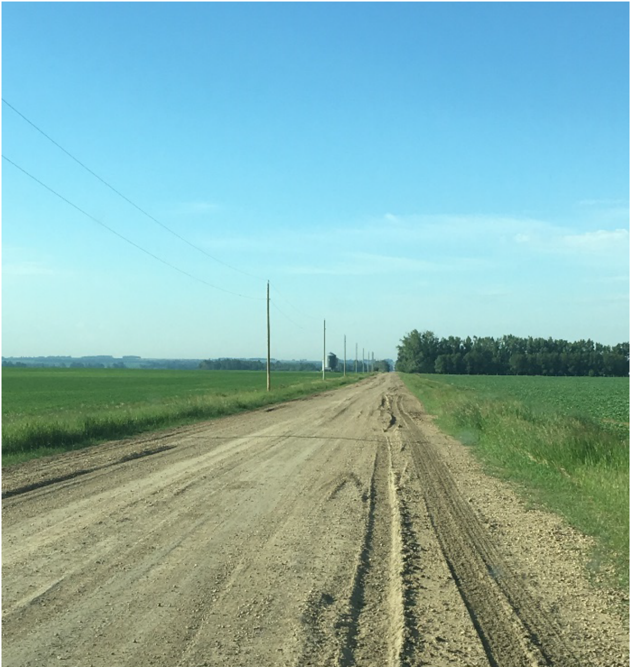
Figure 5-3 - Gravel Road in Moderate Condition (1) – Rating 3.7
