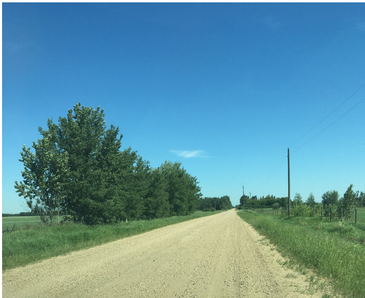
Figure 5-7 - Gravel Road in Good Condition (1) – Rating 4.6
