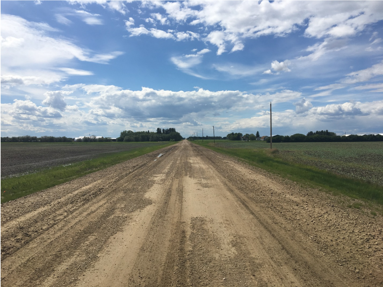
Figure 5-6 - Gravel Road in Moderate Condition (4) – Rating 4.3
