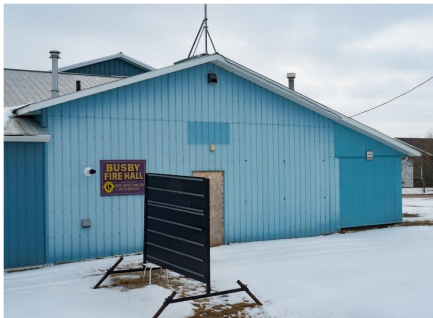
Figure 17 - Busby Fire Hall
