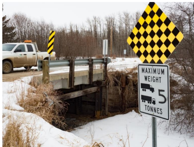
Figure 15 - Local Bridge with Weight Restriction Signage
